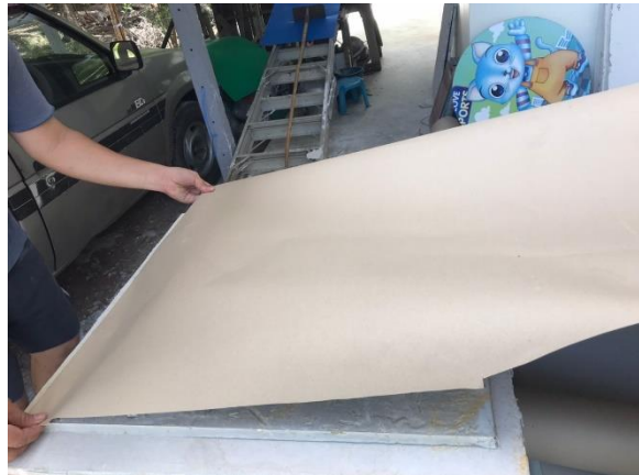
Figure 4 Gypsum board paper installation.
